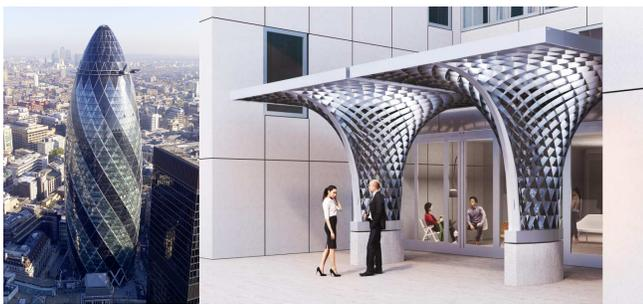
Fig. 2. Principal symmetric meshes in architecture. *Left*: Swiss Re Tower, London, by N. Foster and K. Shuttleworth, *Right*: Canopy for a hotel in Ingolstadt, Germany, by E. Schling and J. Schikore.
