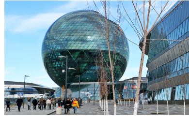
Fig. 19. Spherical glass panels are used by one of the largest spherical buildings in the world, the Nur Alem sphere in Astana, Kazakhstan.
