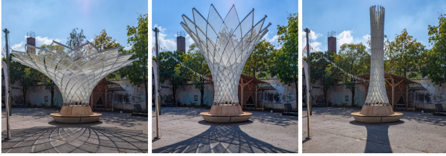
Fig. 2. The 2021 “kinetic umbrella” by Jonas Schikore and Eike Schling is an elastically transformable lattice structure manufactured from straight lamellas. (© J. Schikore).
